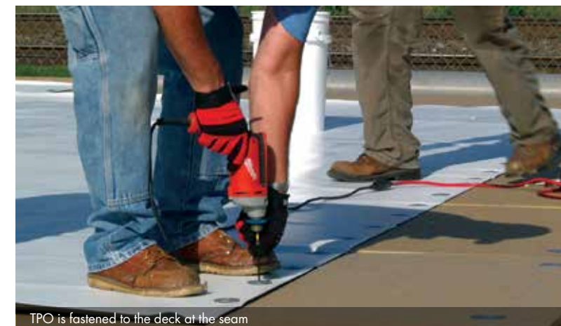
TPO is fastened to the deck at the seam
