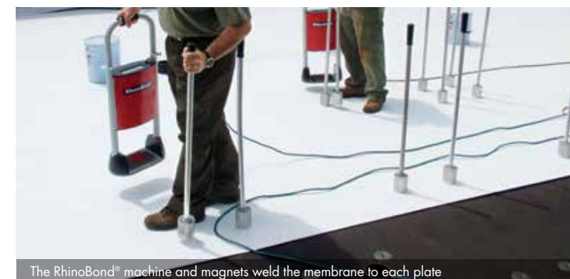
The RhinoBond® machine and magnets weld the membrane to each plate
