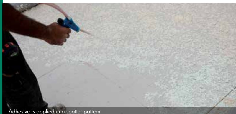
Adhesive is applied in a spatter pattern
