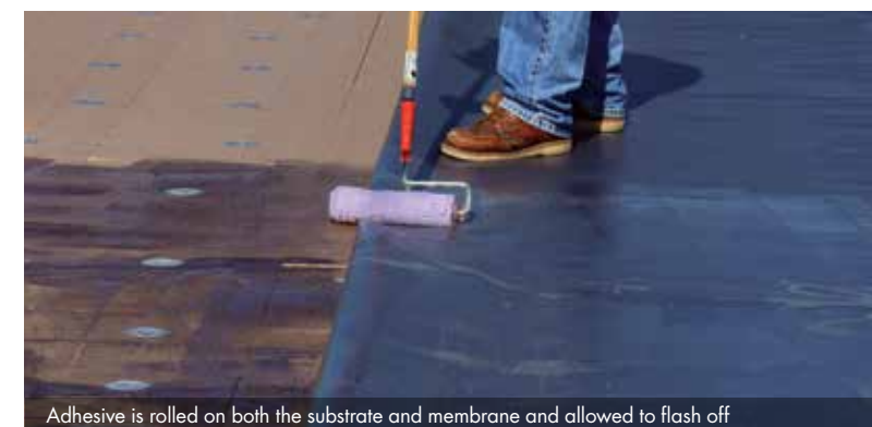
Adhesive is rolled on both the substrate and membrane and allowed to flash off
