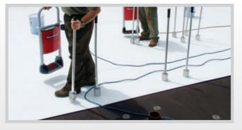
TPO in as low as 25°F (-3.9°C) with LRF M Low Temperature Adhesive. Visit www.gaf.com/tpoinstall for more information on TPO systems.
